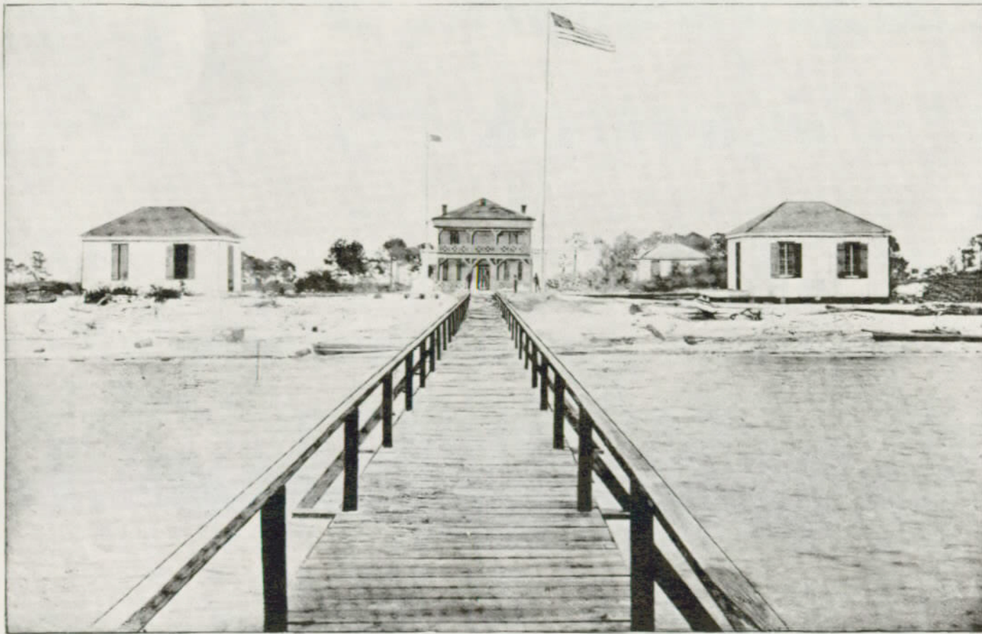
EXECUTIVE BUILDING, U. S. QUARANTINE STATION, SHIP ISLAND, MISSISSIPPI. (VIEW 4.)
