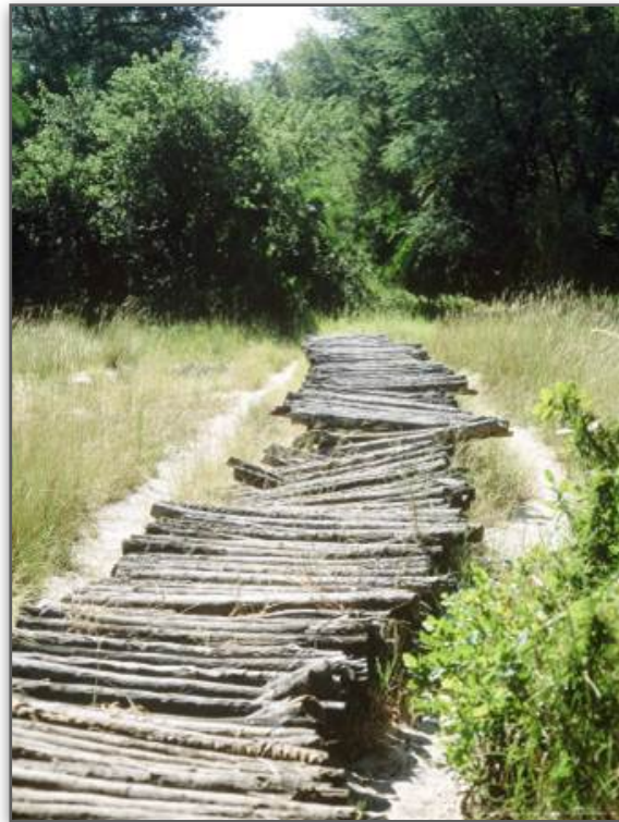
Example of a corduroy road 2
