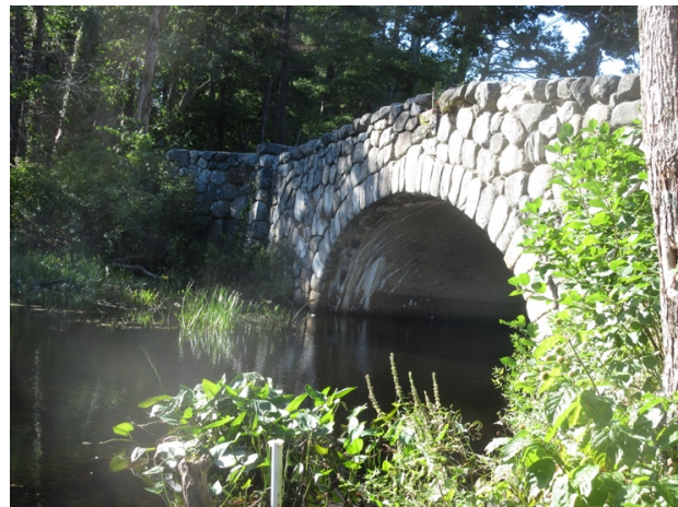
Mile Brook Bridge
